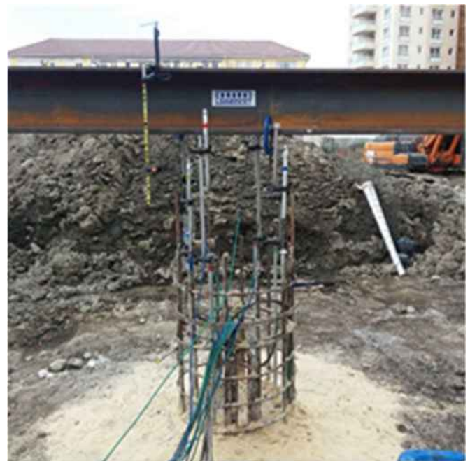
O-Cell® test in progress. The steel beam is for reference only
