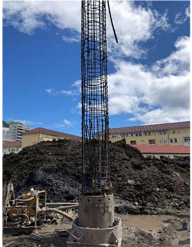
Reinforcing cage, O-cell® and instrumentation being installed into the pile bore
